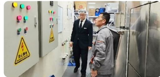
Third-Party Safety Inspection
